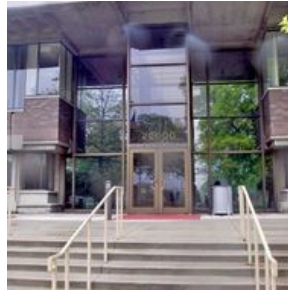
City: Building conditions are not immediate threat to health SOUTHFIELD
