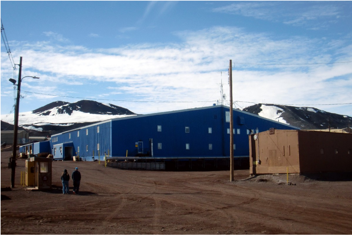
Outside view of building 155, where Armando lodged while in McMurdo.
