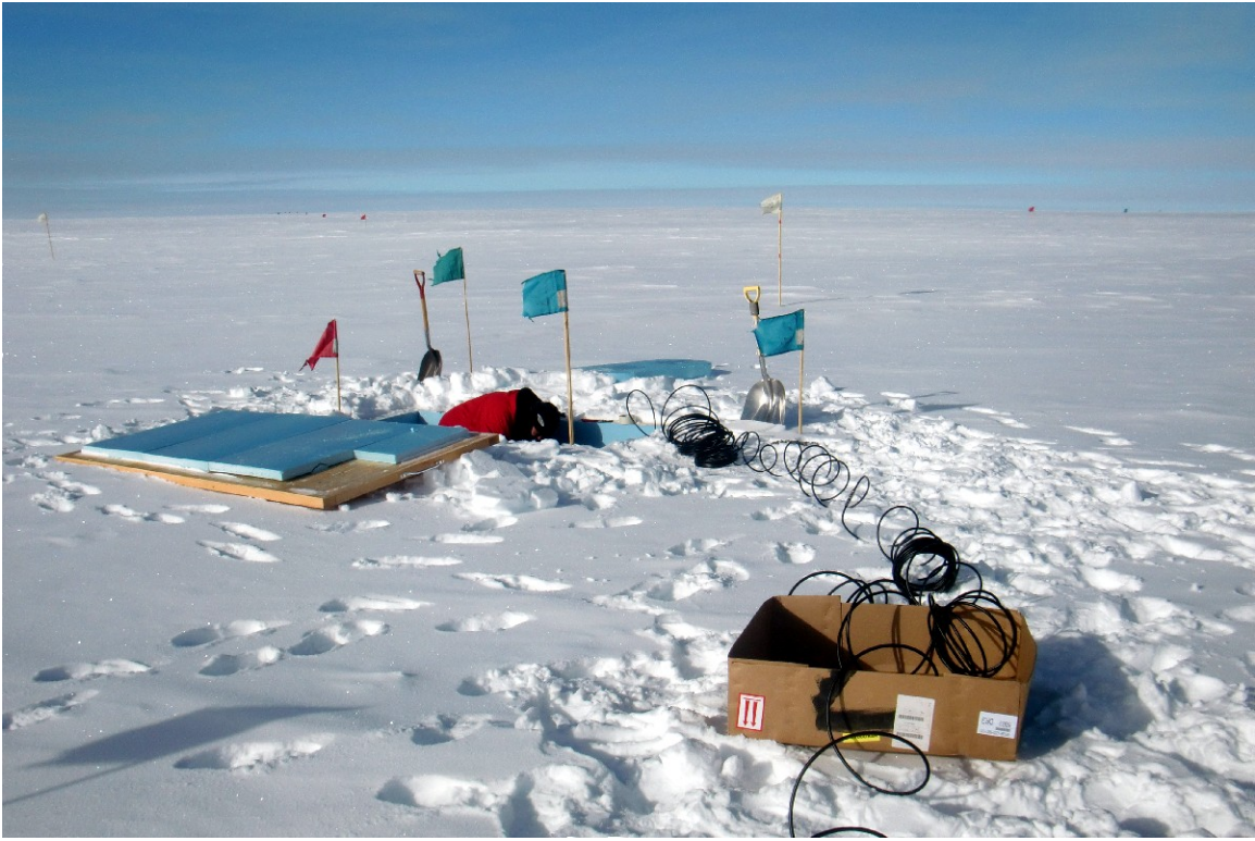
Temporary cabling was installed in order to do tests from 5, 10, 20, 30 and 50 meters away.
