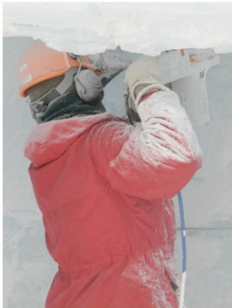
Tim chainsawing the ceiling of the tunnel
