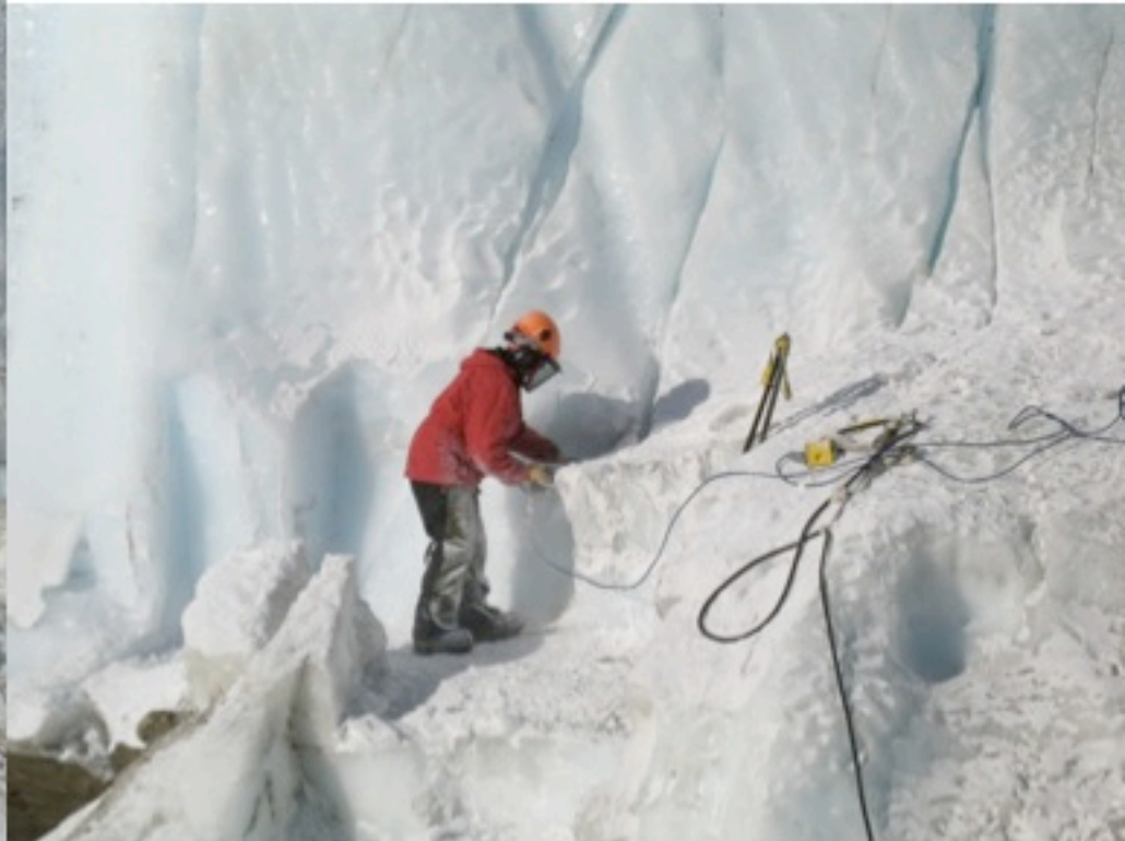
Chainsawing the Start of the Tunnel
