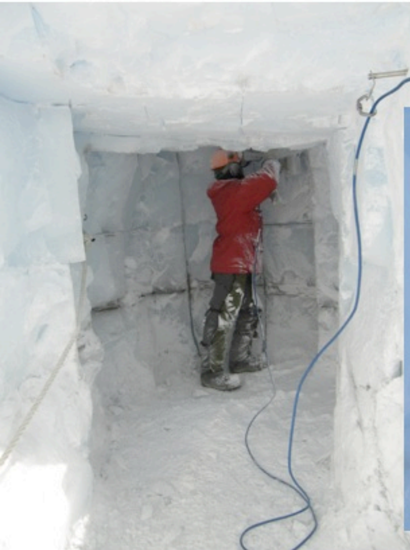
Extending the Length of the Tunnel
