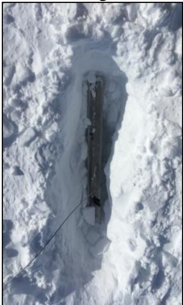
A photo of a deadman that will act to stabilize the AWS tower.
