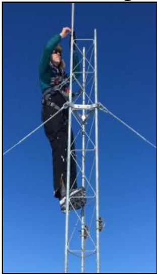
Carol installing sensors on the AWS tower.
